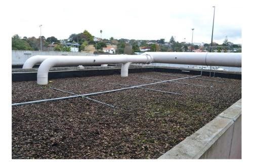
Photo 3: Bio-filter located at the Project Hobson Pump Station
