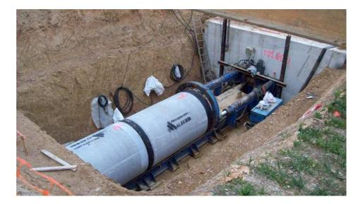
Photo 2: Precast concrete jacking pipes
